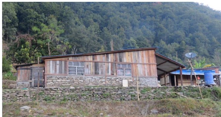
House rebuilt in Lamjung following the earthquake
